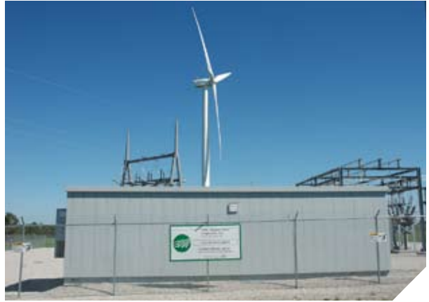
WIND FARM CONTROL BUILDING PROJECT IN GENTRY COUNTY, MO
