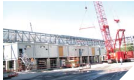
COAL-FIRED POWER PLANT FSG PROJECT IN COFFEEN, IL
