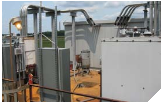
POWER PLANT PROJECT IN MT. VERNON, IN
