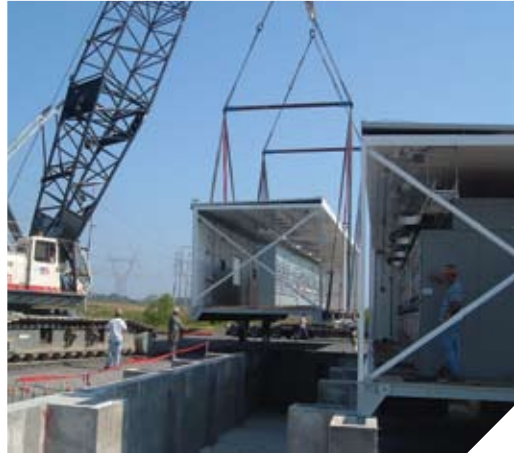
STEEL MILL PROJECT IN DECATUR, AL
