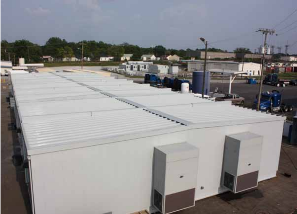
9-Piece, 40ft X 126ft Equipment Center for Coal-Fired Power Plant in St. Charles County, Missouri (included 170 tons of steel and galvanized sheet metal, 350 gallons of paint, 11 miles of wire, over 3,000 points of control wiring terminated, and 110 sections of customer-supplied equipment set, bolted, bussed and interconnected)
